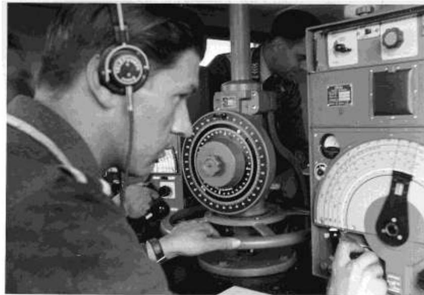
**Interior: Operator at EP2a RX (75 kHz - 3.3 MHz).**
